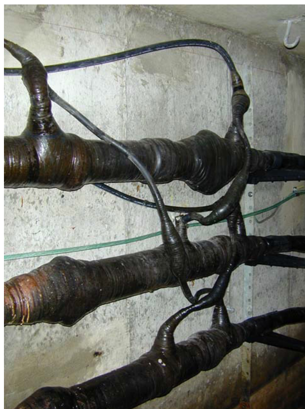
Figure 3. 120 kV sectionalized joints in a manhole
