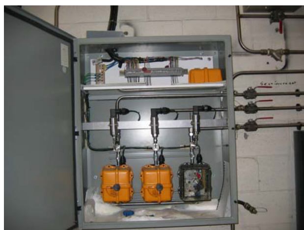
Figure 4. Automated oil pressure monitoring system.
