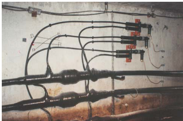
Figure 5. Cross bonding system in a manhole.
